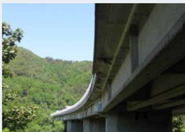
Pecetti Viaduct | ASPI Genova, Italy Assessment and Retrofit
