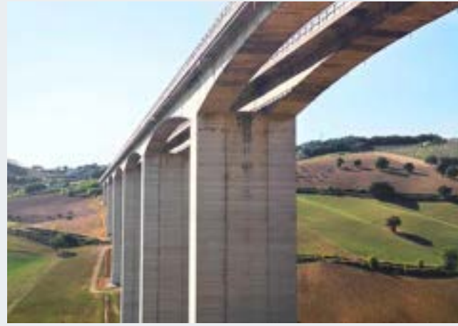
Cerrano Viaduct | ASPI Teramo, Italy Assessment and Retrofit
