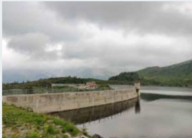
Framework Agreement (20 Dams) | Enel Green Power Italia , Italy Seismic Assessment
