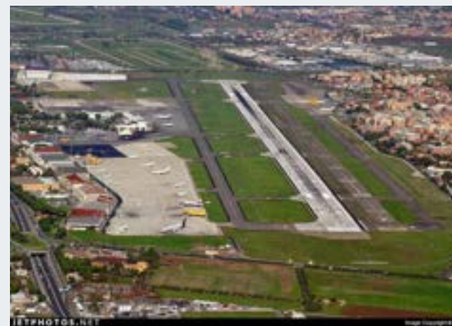
Aeroporto GB Pastine | ADR Ingegneria Ciampino, Italy Static and seismic vulnerability assessment
