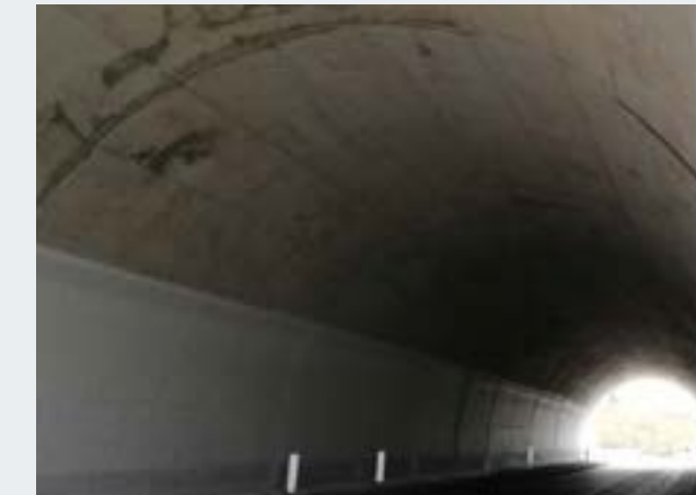
Santa Rufina Tunnel | ANAS Rome, Italy
