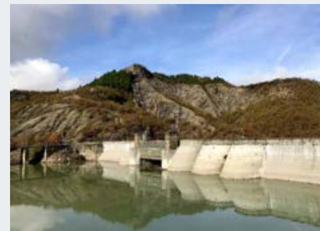
Framework Agreement (40 Dams) | Enel Green Power Italia , Various Locations, Italy Seismic Assessment
