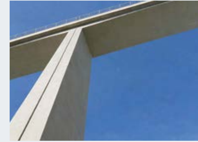
Sori Viaduct | ASPI Genova, Italy Assessment and Retrofit
