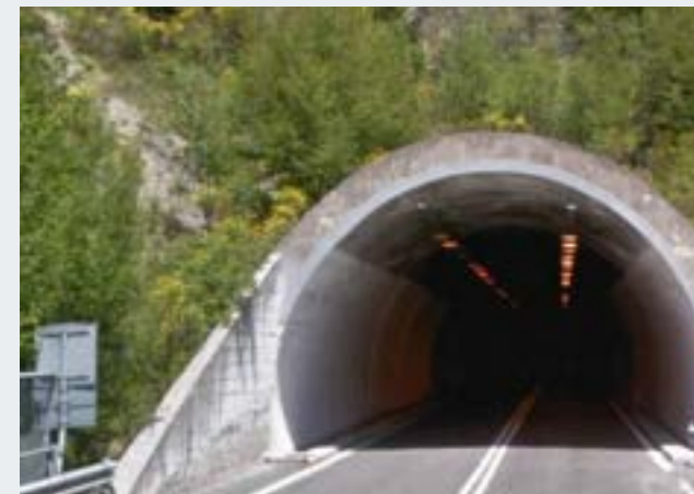
San Pietro Tunnel | ANAS Rome, Italy
