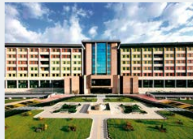
Frosinone Hospital | Local ASL Frosinone, Italy
