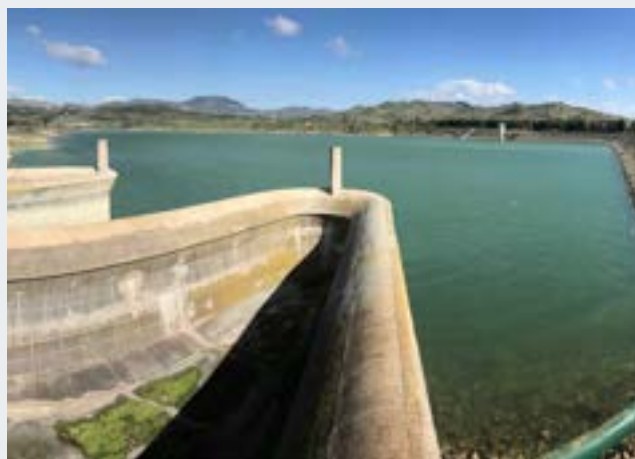
Cimia Dam | Regione Sicilia Niscemi, Italy Seismic Assessment
