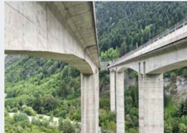
Montbardon Viaduct | RAV A5 Aosta, Italy Assessment and Retrofit
