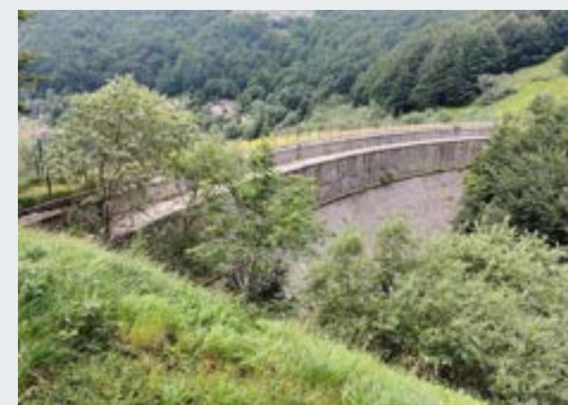
Ballano and Verde Dam | Enel Green Power Italia , Parma, Italy Dam Rehabilitation Design
