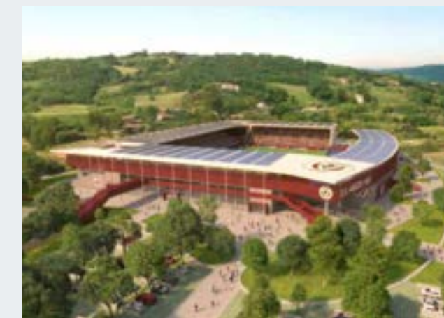
Arezzo Football Stadium | Comune di Arezzo, Arezzo, Italy
