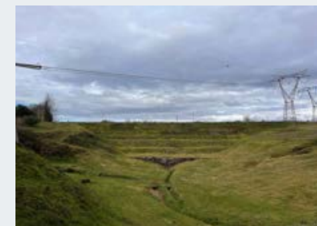
Collemezzo Dam | Enel Green Power Italia Collemezzo, Italy Dam Rehabilitation Design
