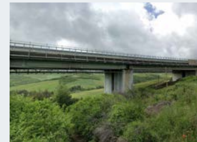
Lamia Viaduct | ASPI Lacedonia, Italy
