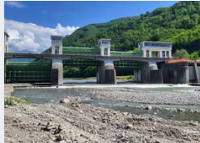
Borgo a Mozzano Dam | Enel Green Power Italia , Lucca, Italy Site Supervision
