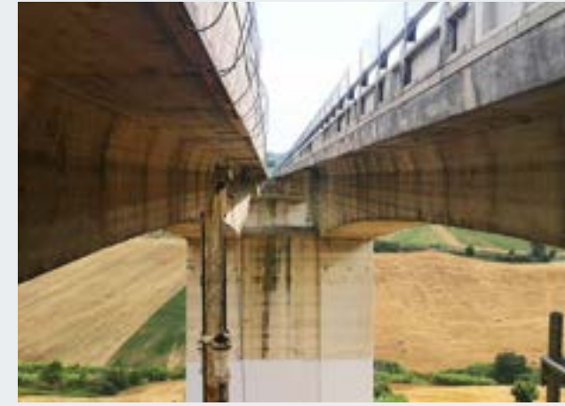
~ 1.000 Bridges | Various Clients Various Locations, Italy Due Diligence and Inspection
