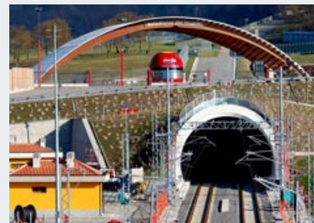
Underground Solutions** | FIAT Bologna - Florence, Italy Geological Works Supervision
