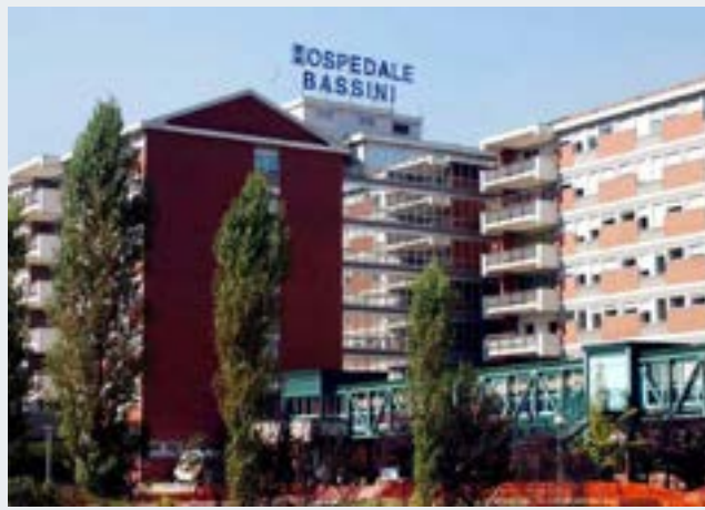
Edoardo Bassini Hospital | Asst Milano 2 Milan, Italy
