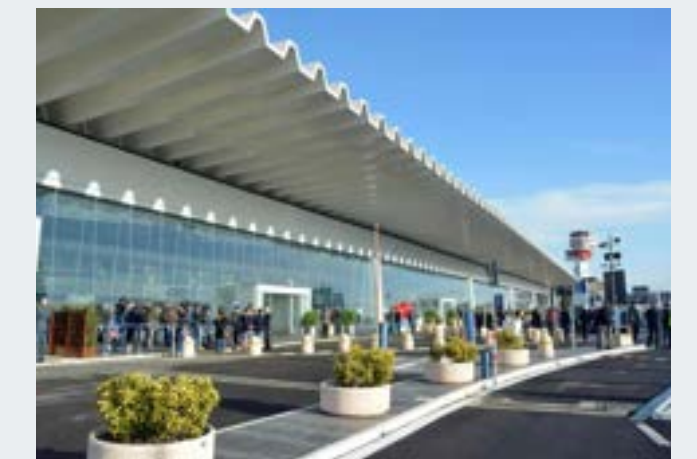
Terminal 3 | ADR Ingegneria Rome - Fiumicino Airport, Italy Seismic Upgrading
