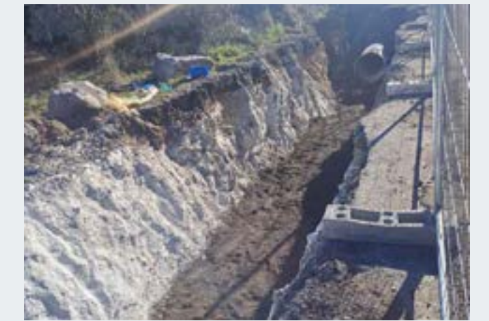
Paschiera New Aqueduct Pipeline | ACEA Monte Castellone, Italy Water System Management
