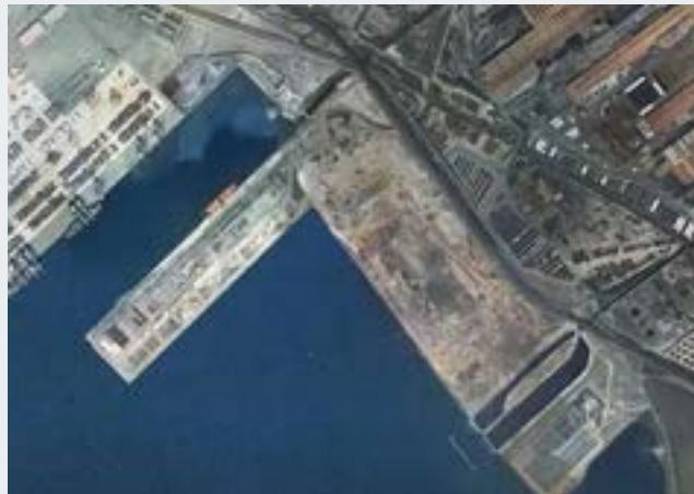
Former Yard Belleli | SOGESID Taranto, Italy
