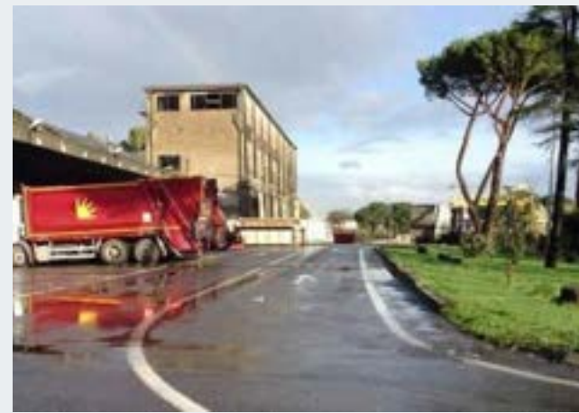
Ponte Malnome Waste Plant | AMA Rome, Italy BIM Construction Management
