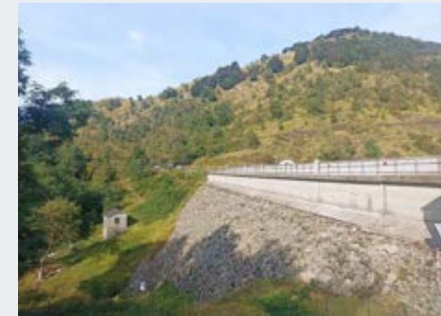
Santa Maria del Taro Dam | Tirreno Power Parma, Italy Seismic Assessment
