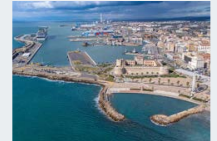
Cold Ironing | ADSP Civitavecchia, Italy
