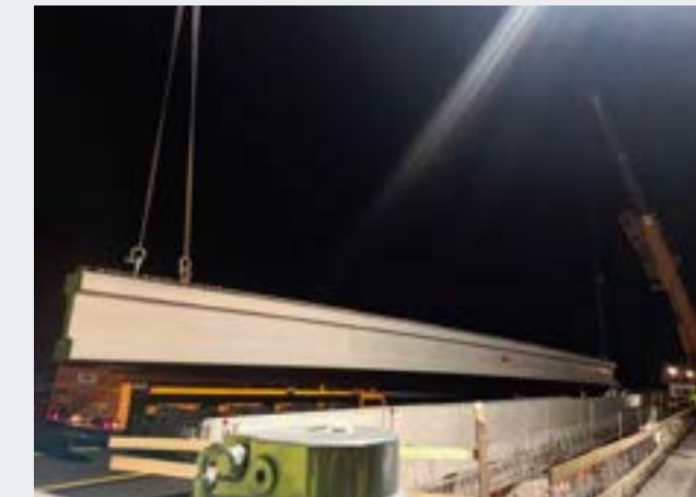
Bridge Crostolo Stream | Autostrade per l'Italia , Italy Assessment and Retrofit
