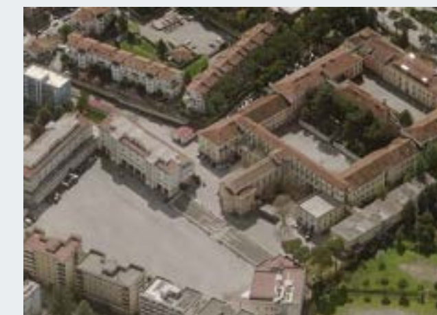
Pepicelli Federal Building | Agenzia del Demanio, Benevento, Italy
